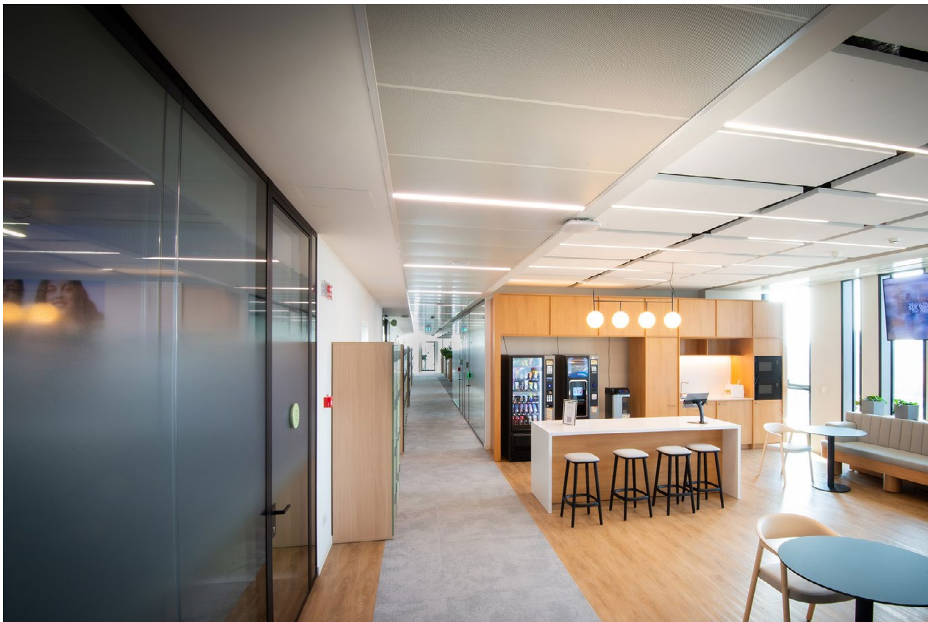
Free-standing tiles, type "C" and "Q" with variable dimensions, Ø2mm perforations and non-woven fabric fleece for increased acoustic comfort.
