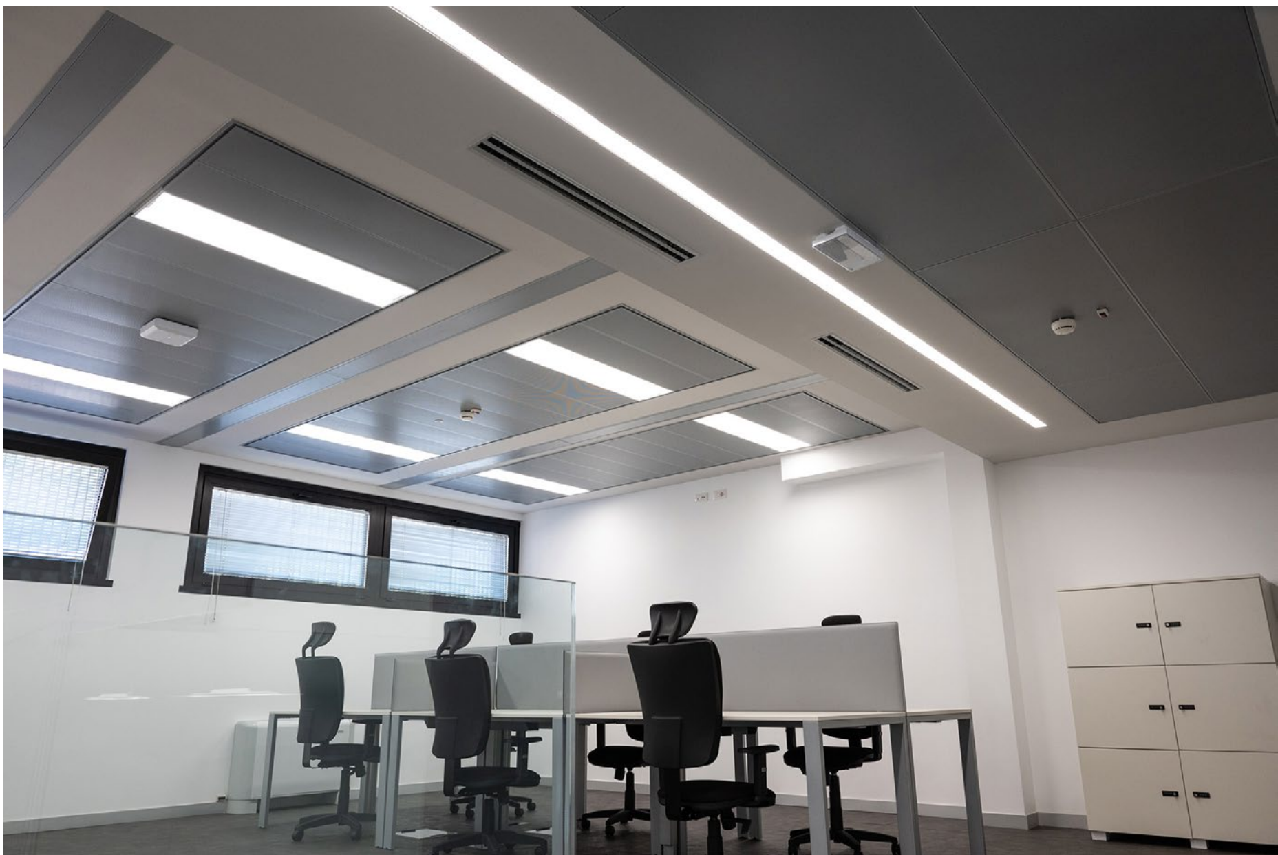
Vert Semi Visio 300x1200 mm and Vert Occulto 600x1800 mm in post-painted silver galvanised steel, micro-perforated and with integrated lighting.
